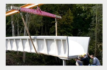
The textile concrete bridge is the second of its type and has double length of its predecessor model in the Saxon city of Oschatz.
