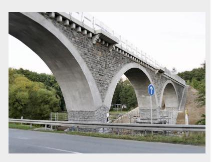
After an elaborate examination of all the available redevelopment techniques, the arches were repaired using carbon reinforced concrete, due to its clear advantages. Two layers of carbon grid were installed and covered using spray concrete lining. The thickness of the carbon concrete was only 20 mm in total, which would not have been remotely possible with steel reinforced concrete.
