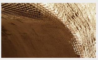
The existing cracks were pressed, and the previous cross-section was reprofiled under the specifications to maintain the previous cross-section. For reinforcement, 2 layers of carbon reinforcement with spray concrete with a total thickness of 20 mm were incorporated.
