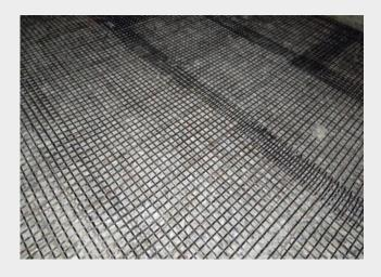
For restoring durability, an additional layer of concrete was required in order to create a gradient. Due to the low ceiling height of the garage, a carbon reinforcement was used instead of a conventional steel reinforcement. The carbon grid structure was placed close to the surface and covered with a 20 mm concrete layer. A gradient of 2.5% was also incorporated
